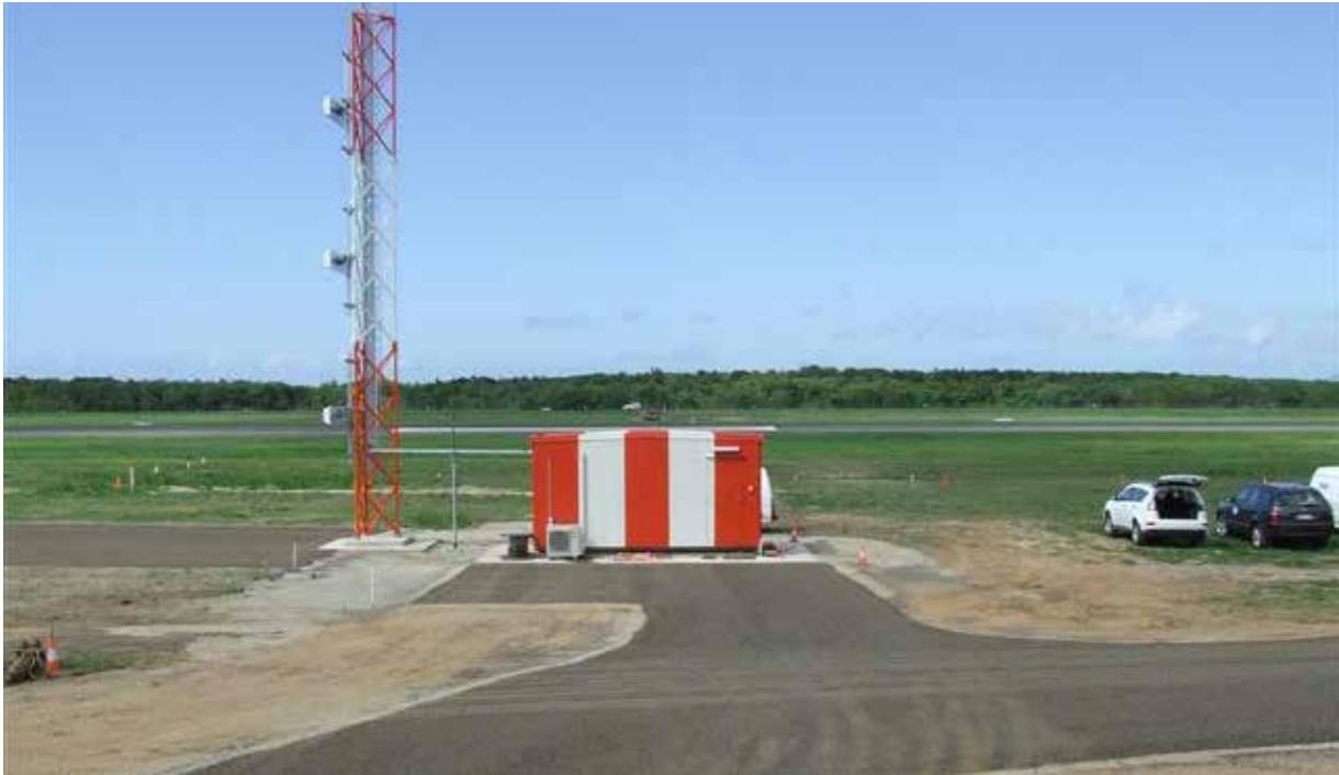
Figure 2.2: Typical Glidepath Installation
