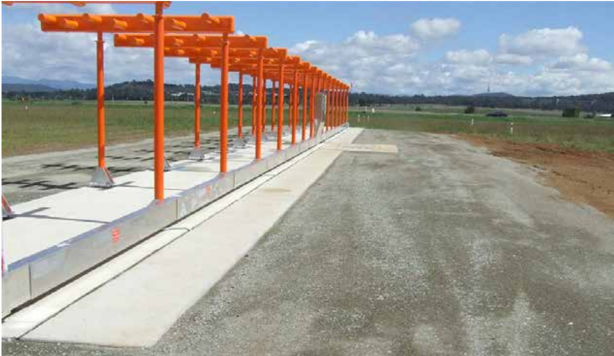
Figure 2.1: Typical Localiser Installation
